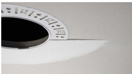
Partially finished mud ring, showing cross-section detail.
