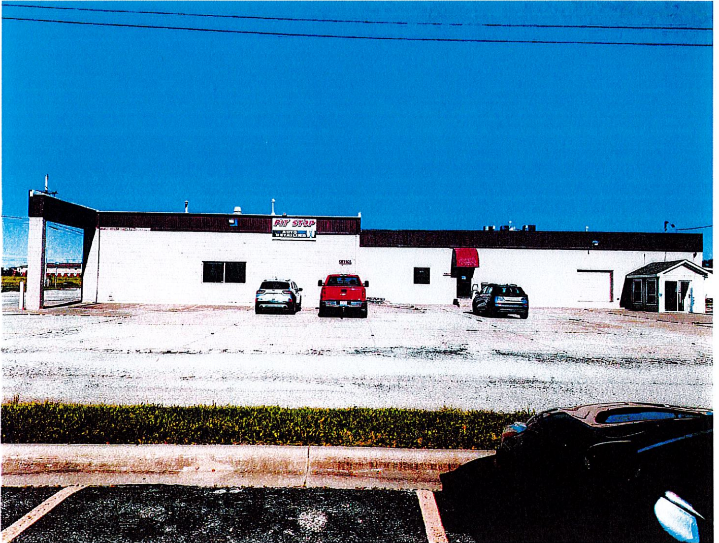
East side of Property
