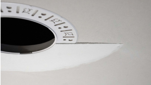
Partially finished mud ring, showing cross-section detail.
