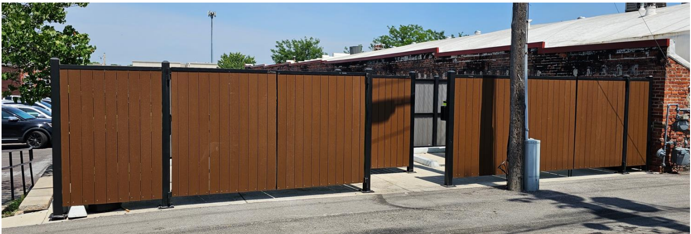
Figure 2 – Trash Enclosure at 216/218 SE Douglas St
