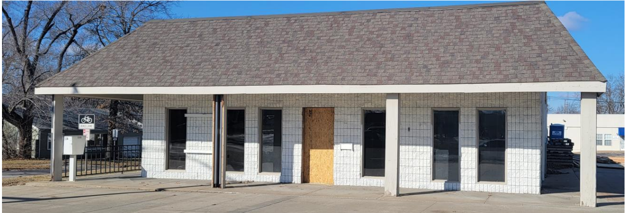
Figure 2 – Existing south façade of the subject building
