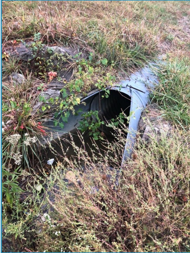
Figure 6 - Detention Basin Outlet North of Bowlin Road
