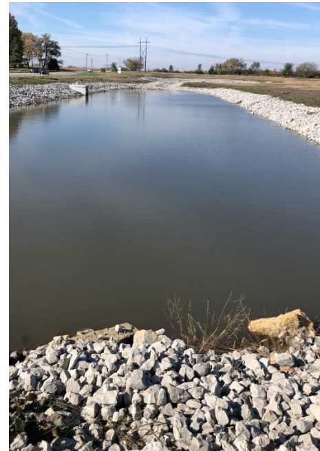
Figure 3: Existing Site Condition (Nov. 05, 2021)
