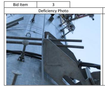
Install cable guides above and below obstructions at 99', 129' and 145' as needed to prevent cable from rubbing on obstruction(s). Install Tuf-Tug step bolt anchor brackets on the (3) existing step bolts above and below the obstruction(s) and all additional step bolts located through the obstruction(s).
