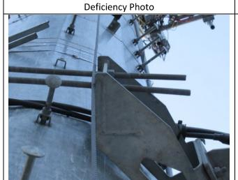
Replace (1) missing step bolt at 104'. Step bolts to be a minimum of 5/8"Ø x 8" ASTM A449 w/ 4.5" unthreaded shank or equivalent.
