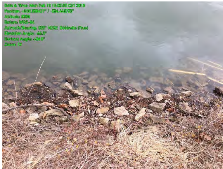
Photo 2- Upstream face rock "erosion control"
