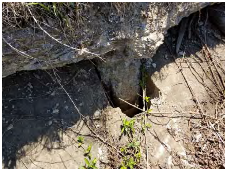
Figure 8: Photograph of Spillway Puncture
