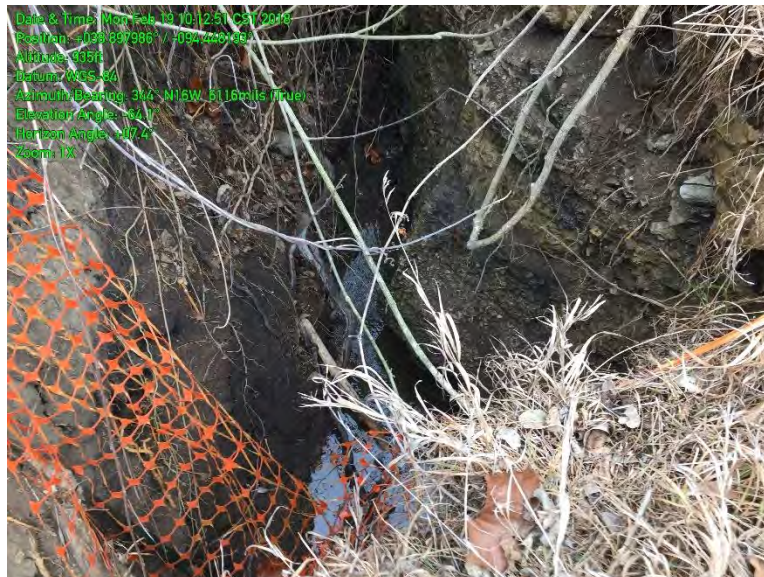
Photo 7- Seepage under emergency spillway
