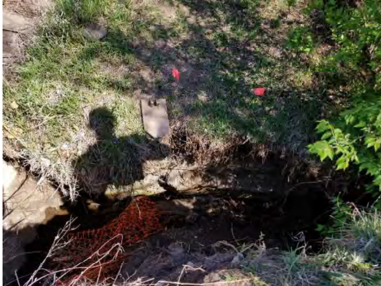
Figure 11: Photograph of Erosion Around West Side of Spillway
