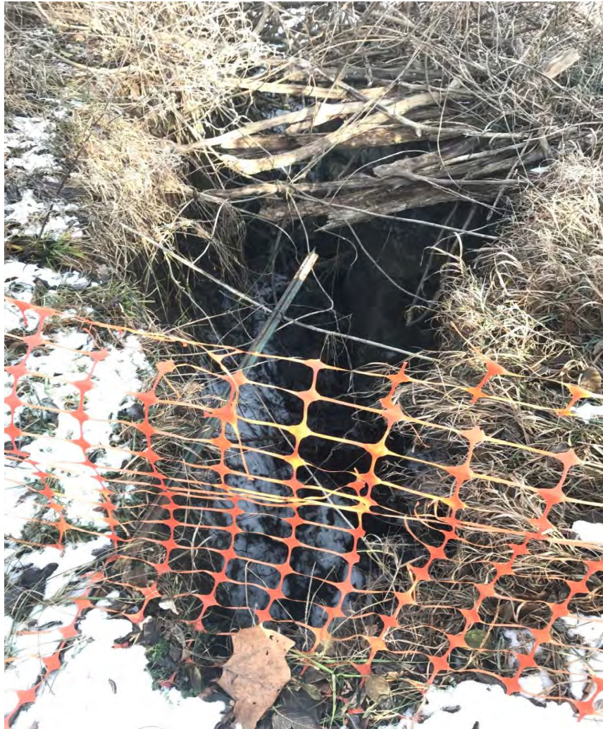
Typical view of erosional channel adjacent to spillway structure.
