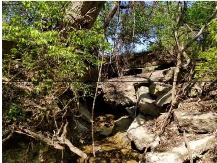
Figure 9: Photograph of Erosion Below Concrete Apron
