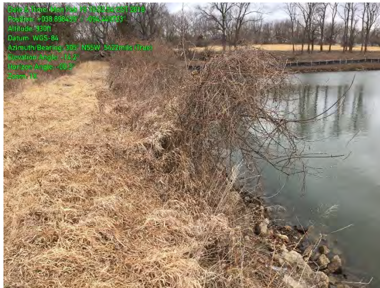
Photo 3- Looking west at freeboard erosion of embankment
