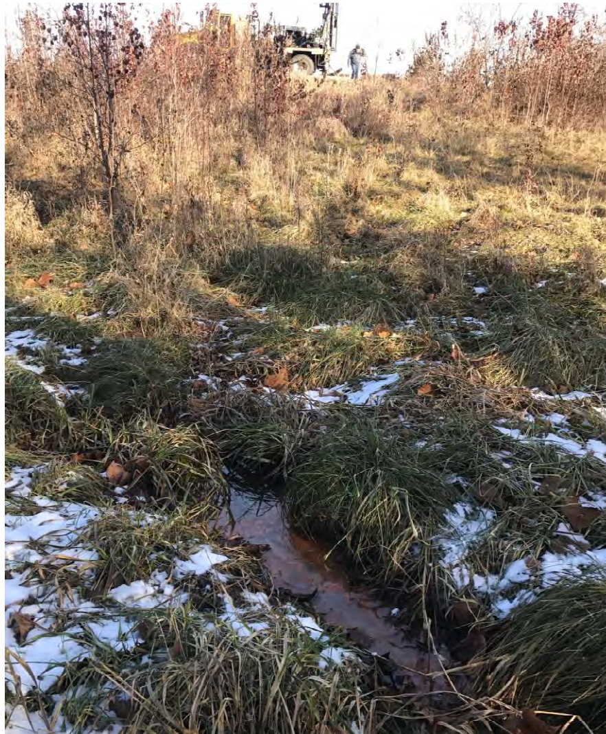
Typical view of water seepage at toe of dam.
