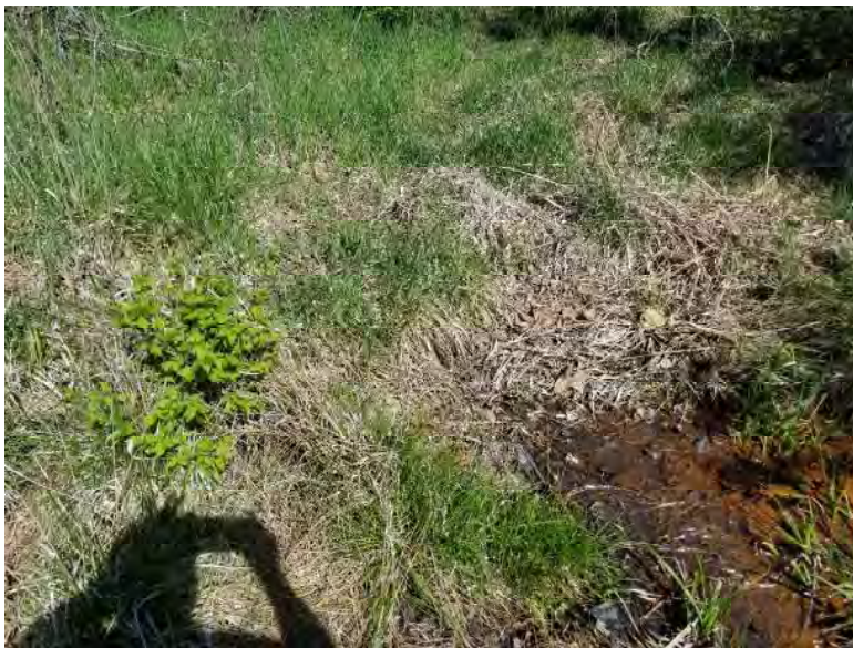
Figure 6: Photograph of Seepage at Toe of Dam
