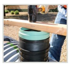
Drive the plastic hub into the rubber sleeves with a 4 pound mallet and block of wood. Stop when the rubber sleeve meets the red line.
