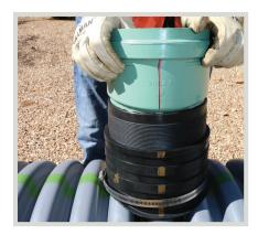
Apply soap solution to inside of the inner sleeve and on the PVC hub. Insert the PVC hub into the sleeve by hand until snug fit, aligning the red line on the hub with the gold lines on the rubber sleeves.
