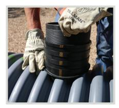
Insert the rubber sleeves into the cored hole, with the gold lines perpendicular to the pipe. Once in place, pull up on the inner sleeve and push down on the outer sleeve until fitted to the host pipe.
