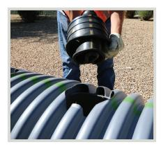
Use the coupon to estimate the separation between the two sleeves and fit the two sleeves together. Be sure the gold lines on the sleeves are lined up.
