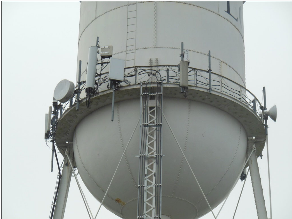
Existing T-Mobile Antennas on Handrail (Typ.)
