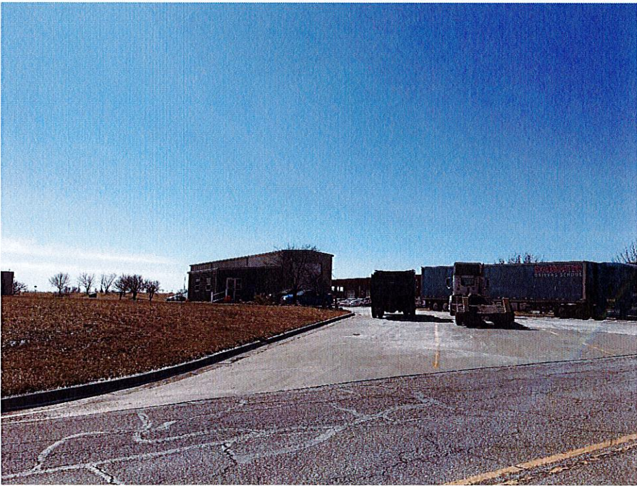
MODOT Service facility south of Town Center Drive
