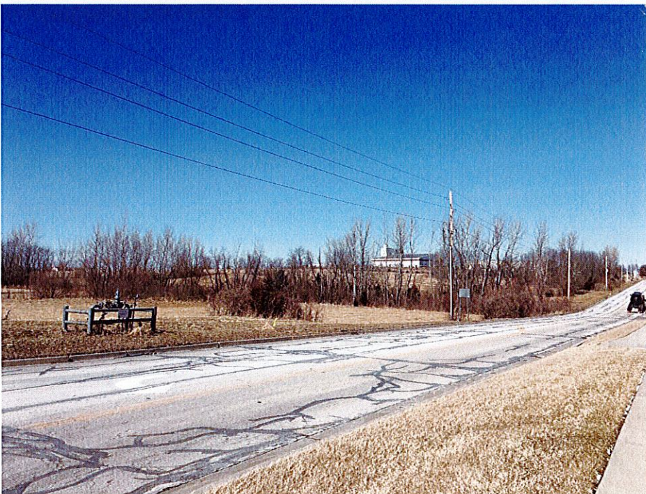
View of property looking northwest from Independence Ave.
