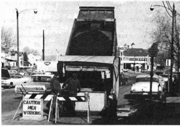
Fig. 2. Truck dumping fill at a flushing hopper.
