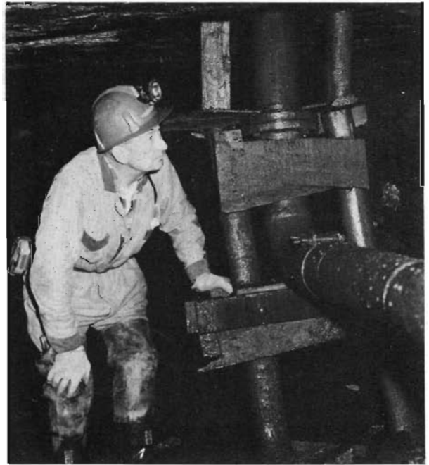
Fig. 5. Elbow at the foot of a controlled flushing borehole.
