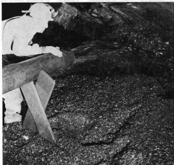
Fig. 7. Slurry flowing from an underground pipeline during controlled backfilling.
