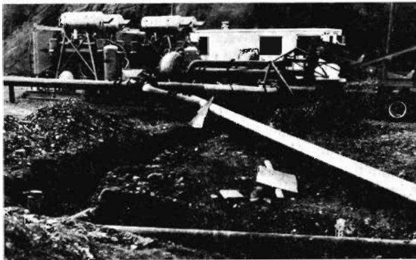
Fig. 9. A pumped-slurry plant; water enters pipe at left; solids enter tank from conveyor at right; suction line transmits slurry to pump in center; slurry enters distribution pipeline that passes under water pipeline to right foreground.
