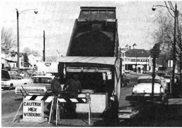
Fig. 2. Truck dumping fill at a flushing hopper.
