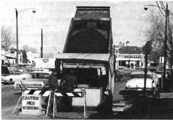
Fig. 2. Truck dumping fill at a flushing hopper.
