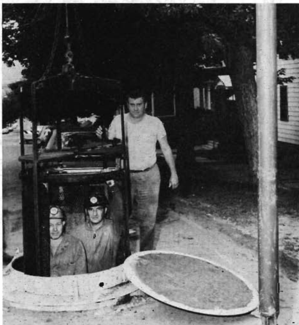
Fig. 4. Hoisting cage for access to the mine workings in a controlled backfilling operation.
