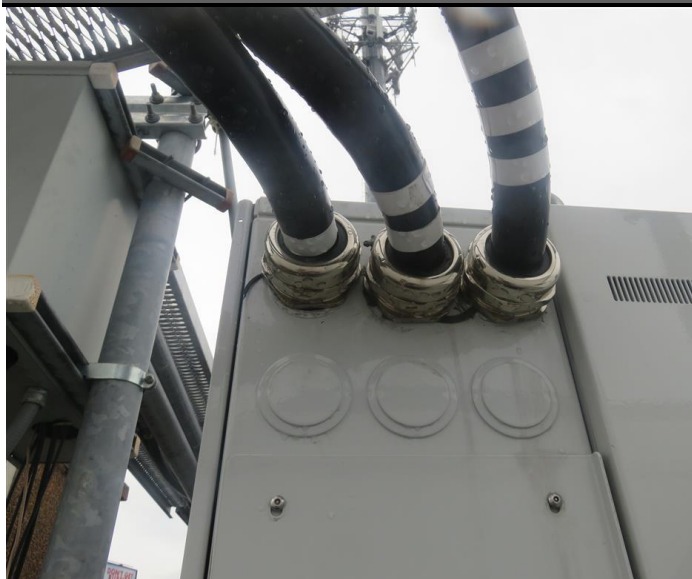
COAX ENTERING CLEARWIRE CAB
