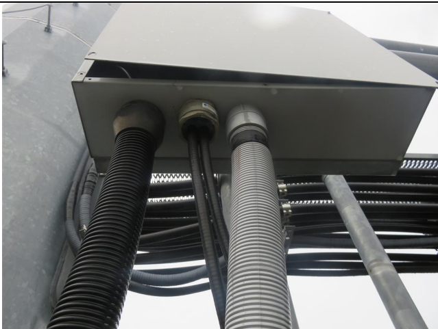
COAX ENTERING CLEARWIRE CAB
