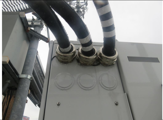
COAX ENTERING CLEARWIRE CAB
