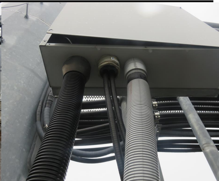
COAX ENTERING CLEARWIRE CAB
