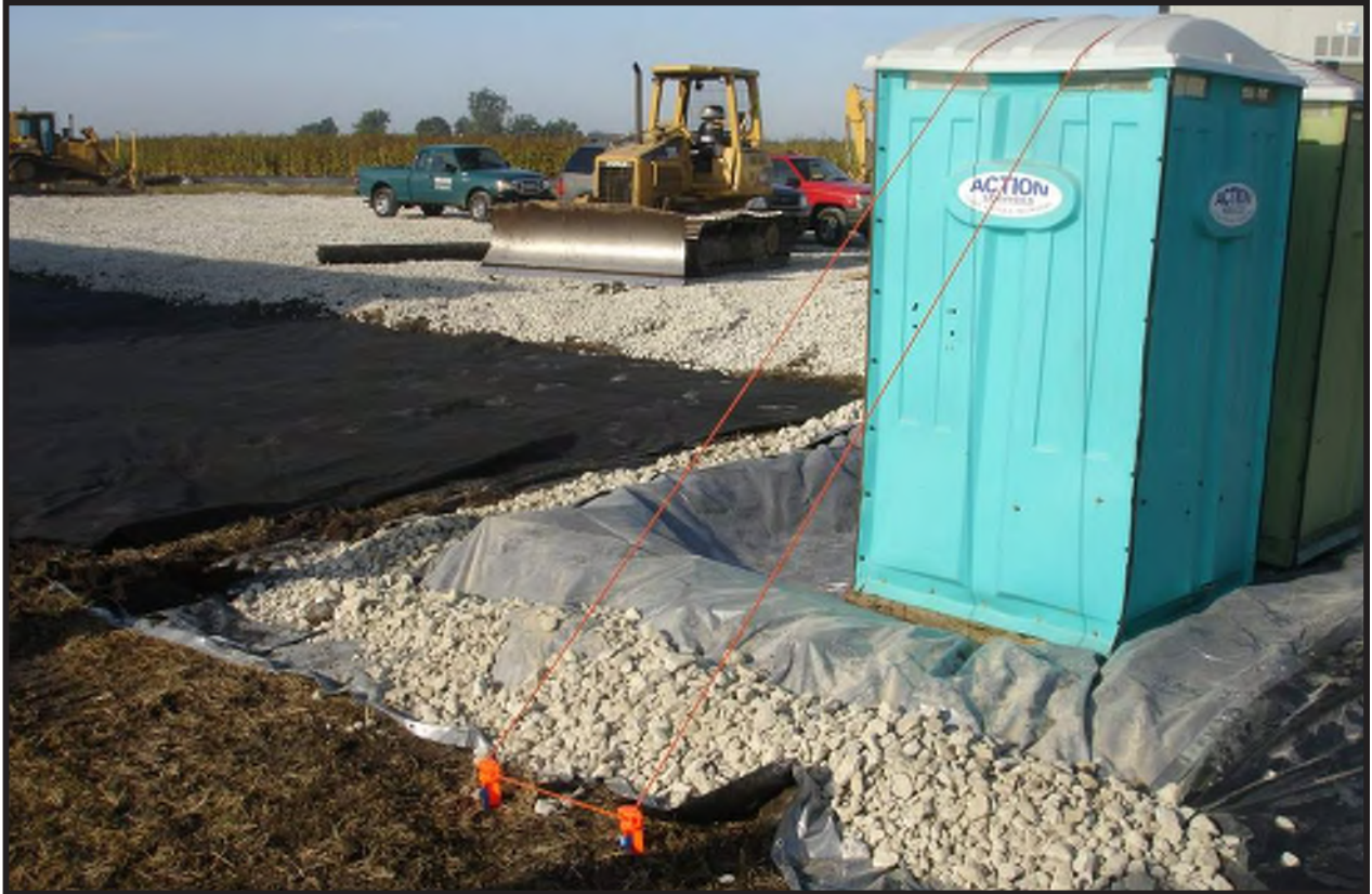
Figure 6.18 Typical port-a-potty with secondary containment and tie downs. Source: BFA Inc.
