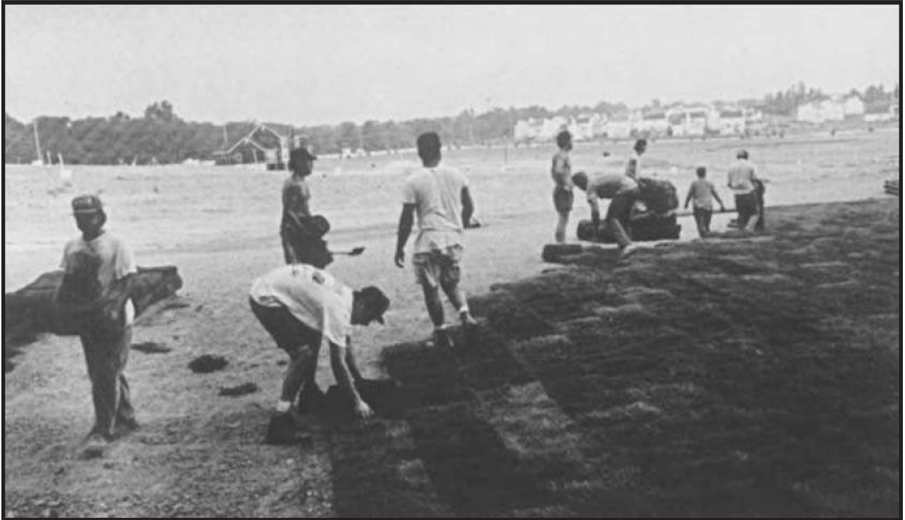
Figure 6.34 A team is laying sod strips so the seams are not aligned and the ends and sides are against each other to reduce drying out of the roots. Source: N. Klopfenstein, NRCS. St. Charles Co.
