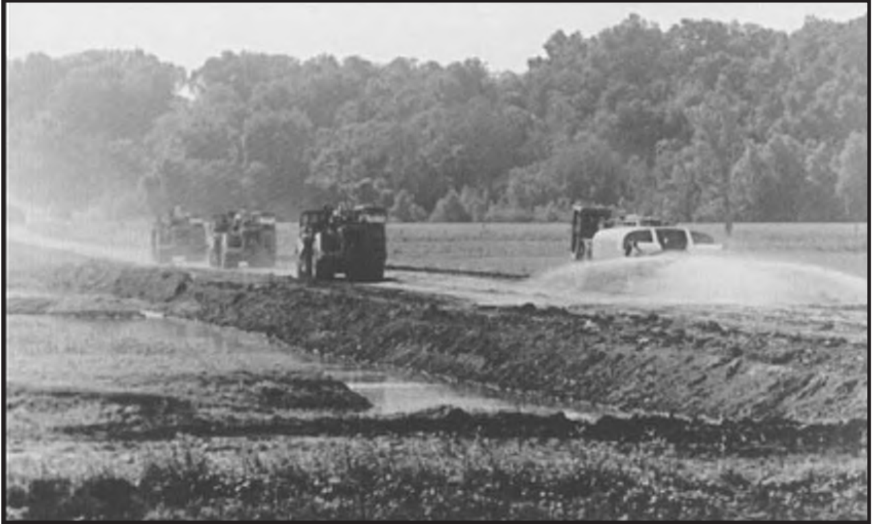
Figure 6.33 Spraying water is effective for dust control on haul roads, although it must be frequently repeated during hot days or heavy traffic periods. Source: C. Rahm, NRCS, St. Charles Co.
