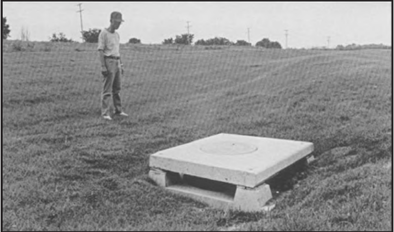
Figure 6.25 Permanent vegetation can be used to stabilize many structures, such as this grassed waterway, ensuring that runoff is relatively sediment-free.
