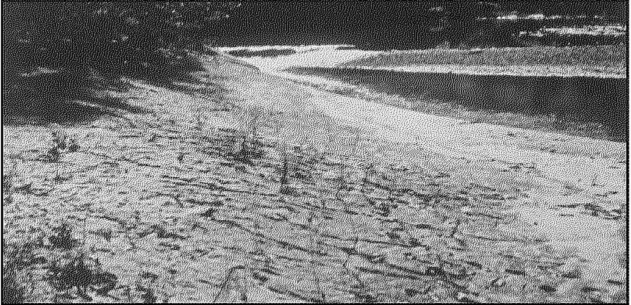
Figure 6.37 Willows and other live stakes will root and sprout rapidly to protect slopes. The roots form an interlocking mat to hold soil in place, while the foliage protects the soil surface. These willows, planted along Hinkson Creek in Columbia, were 3- to 5-feet tall within six months. Source: Doug Wallace. NRCS. Boone Co.
