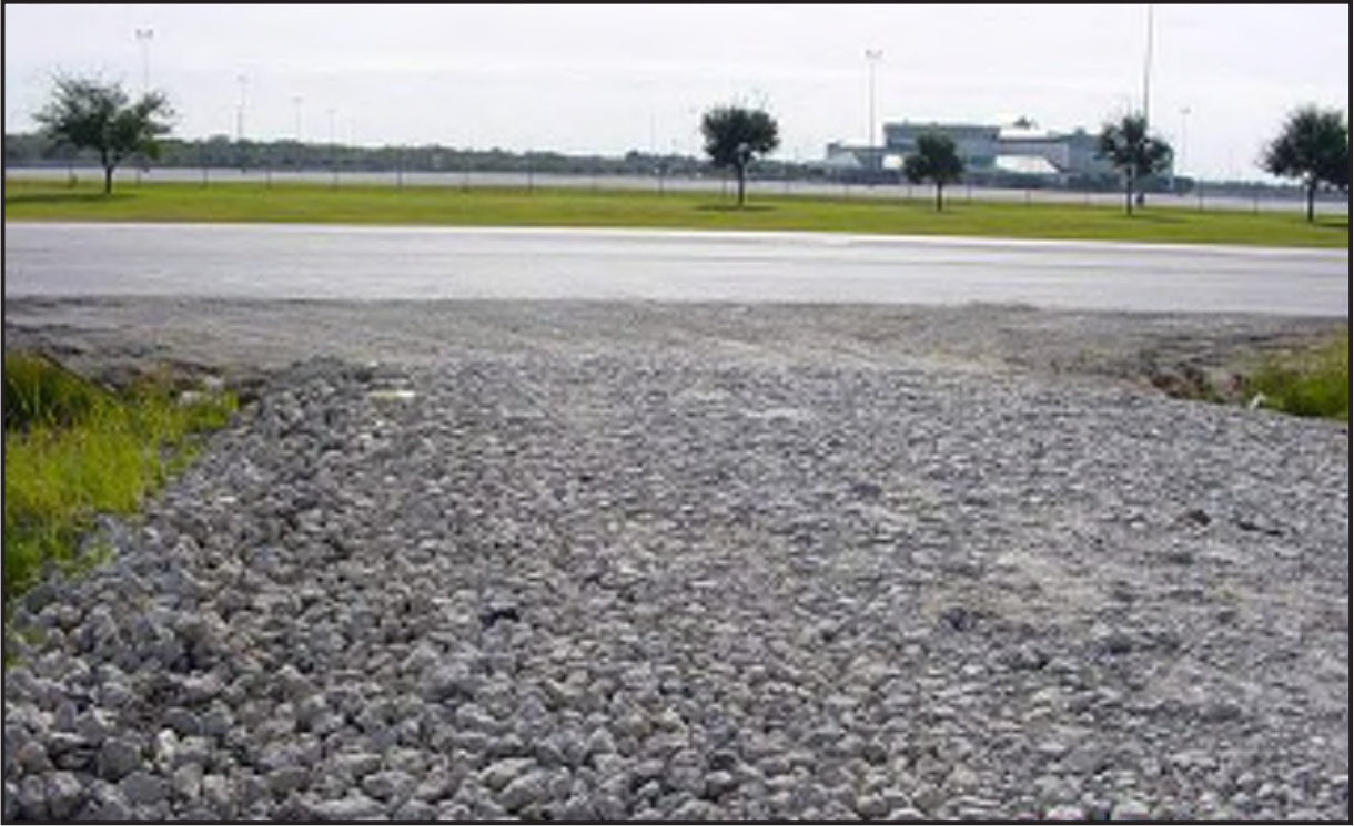
Figure 6.1 A temporary rock construction exit can reduce sediment and resulting safety hazards on public streets. This pad needs maintenance due to sediment filling the void spaces between the rocks making the rock exit pad ineffective. Source: ABC's of BMP's, LLC
