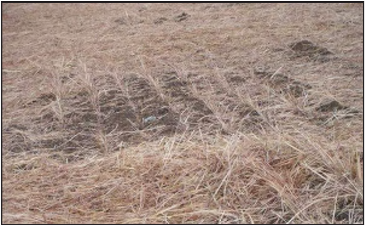
Figure 6.28 Crimped straw. Source: ABCs of BMPs, LLC.
