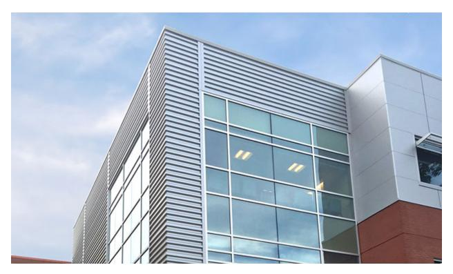
MBCI 7.2 deep ribbed panel horizontally oriented, in a metallic silver finish. Panels used on an office building to create contrast with the adjacent flat metal wall panels.
