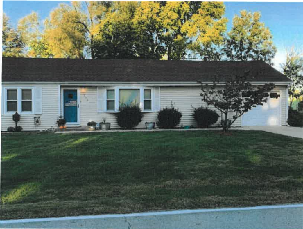
Existing Ranch Style Home
