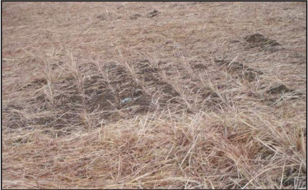
Figure 6.28 Crimped straw. Source: ABCs of BMPs, LLC.
