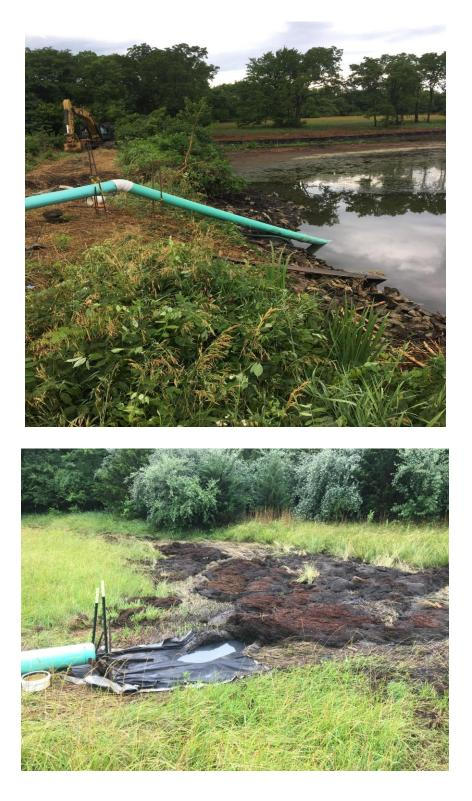
No water was observed flowing over the blanket of the spillway or through the eroded area on the west side of the spillway. Visually, the dam, spillway and erosion channel do not appear to have changed since our initial visit. We have included a current photograph of the area below.
