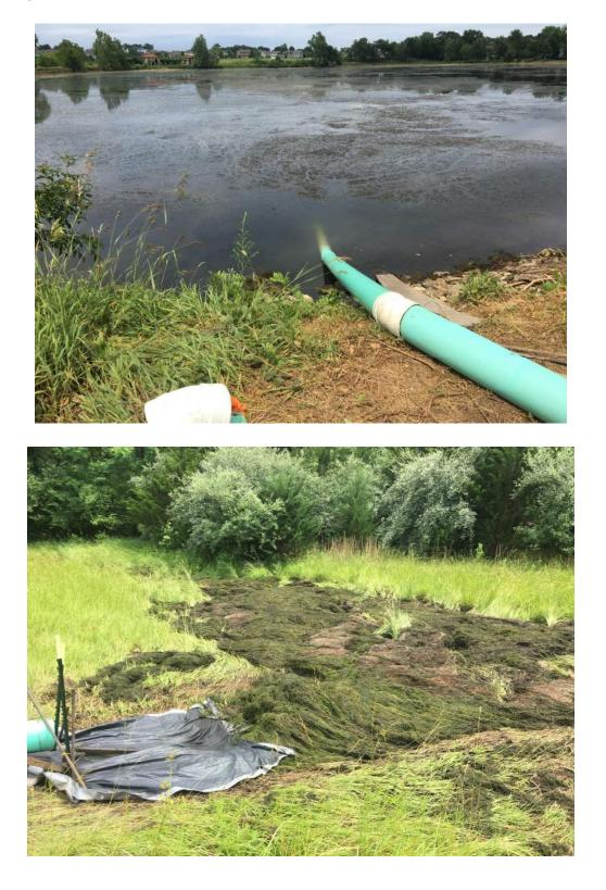
No water was observed flowing over the blanket of the spillway or through the eroded area on the west side of the spillway. Visually, the dam, spillway and erosion channel do not appear to have changed since our initial visit. We have included a current photograph of the area below.
