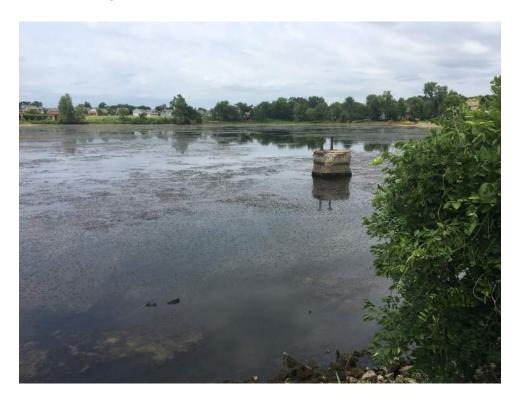
In addition, the pipe was no longer drawing water from the lake due to clogging from vegetation. Moss is shown at the base of the hill where the pipe outlets. This is shown in the Figure below. We understand the water collection area is to be deepened and cleaned in order to continue syphoning.
