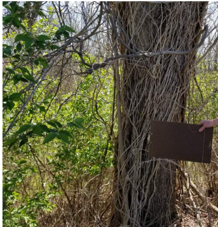
Figure 4: Photograph of Large Mature Tree on Crest of Dam
