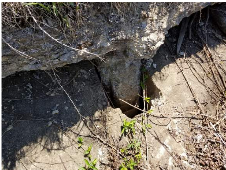
Figure 8: Photograph of Spillway Puncture
