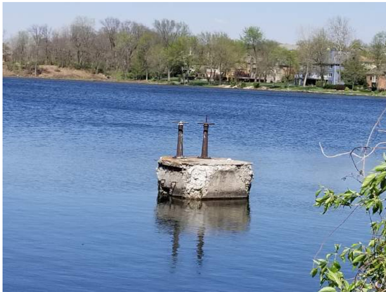
Figure 7: Drawdown Structure
