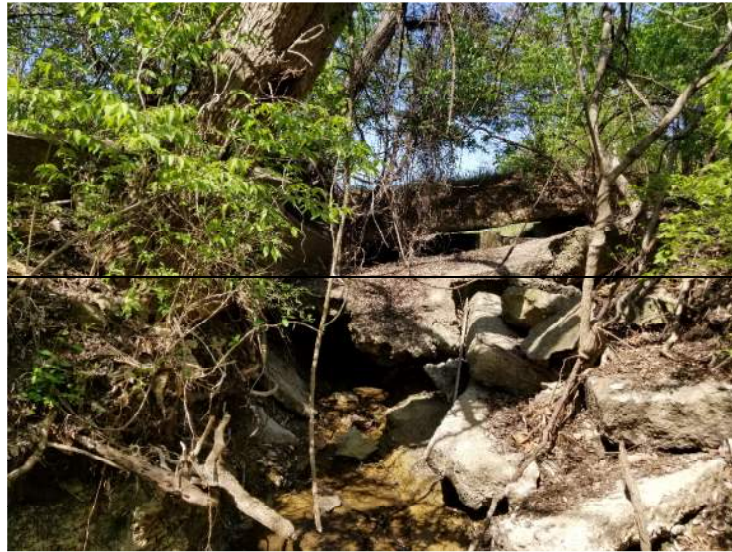
Figure 9: Photograph of Erosion Below Concrete Apron
