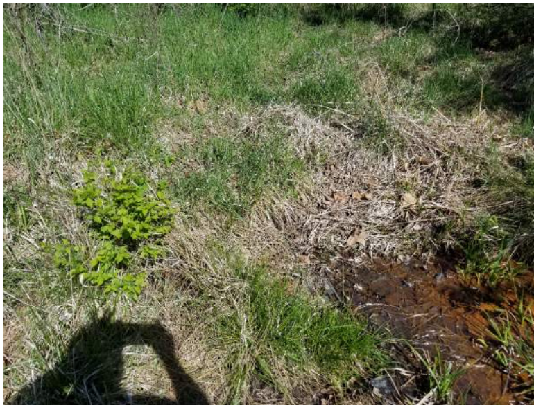
Figure 6: Photograph of Seepage at Toe of Dam
