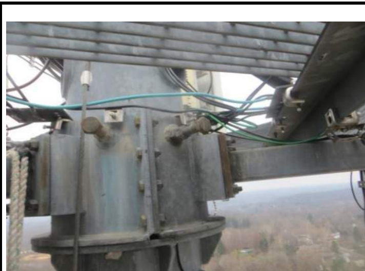
Side Connection at Tower (Level & Perpendicular)
