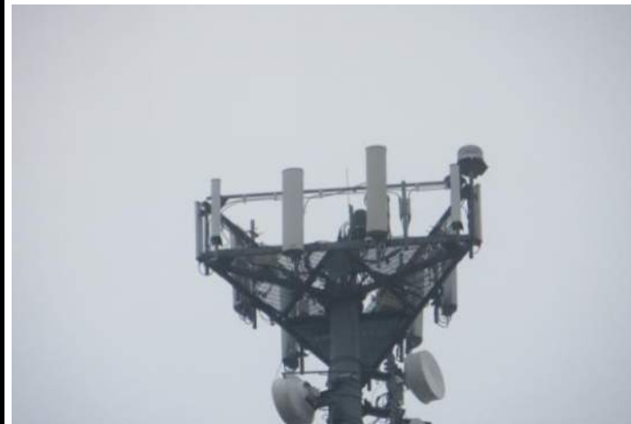
All Booms on Structure (Zoomed in, taken from ground)
