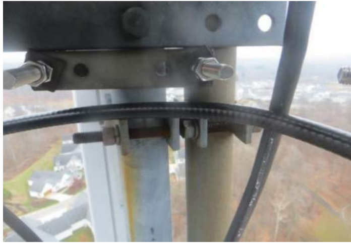
Back Side of Top Connection at Boom (Level & Perpendicular)
