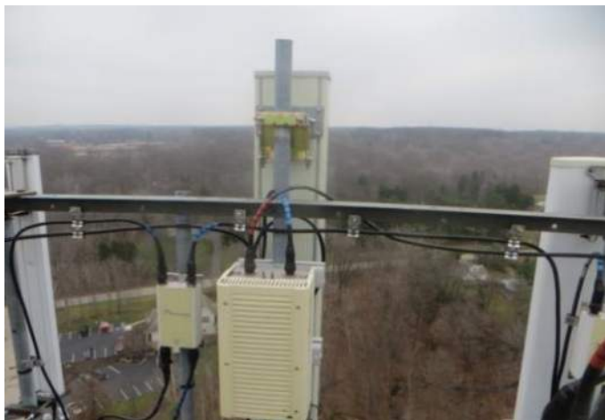
Back Side of Full Ant. #3 (Level & Perpendicular)
