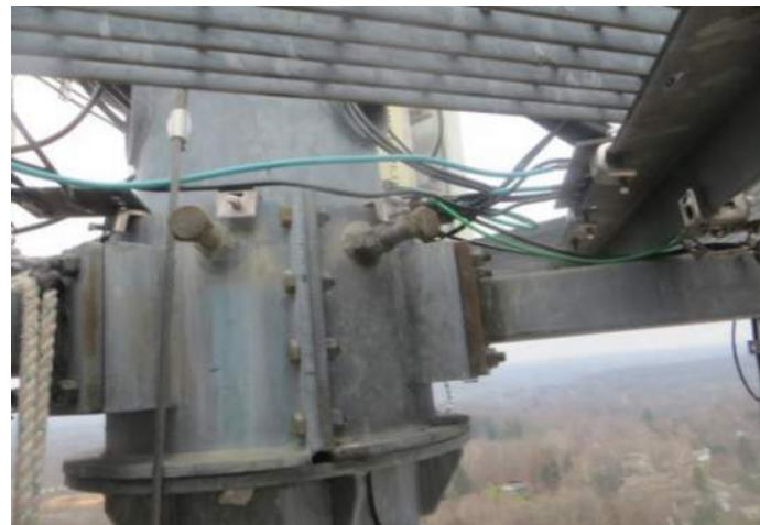
Side Connection at Tower (Level & Perpendicular)
