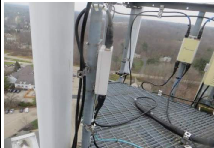
Full Side TMA(s) (Level & Perpendicular)
