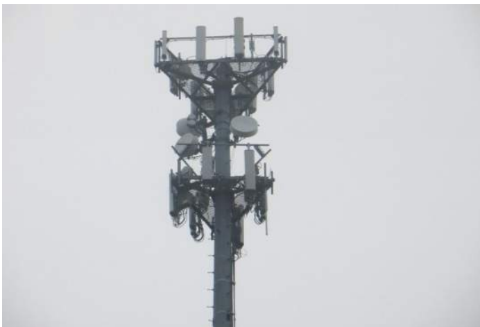
Mount Section - North Face (Entire Section, Taken From Ground)
