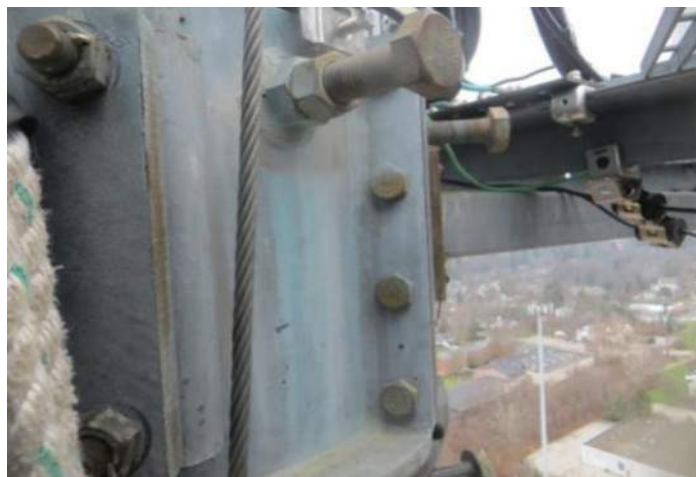
Underneath Collar Mount (Straight Up)
