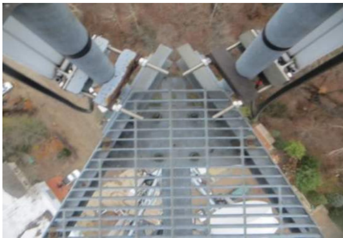
Back Side Connection at Side Arm (Level & Perpendicular)
