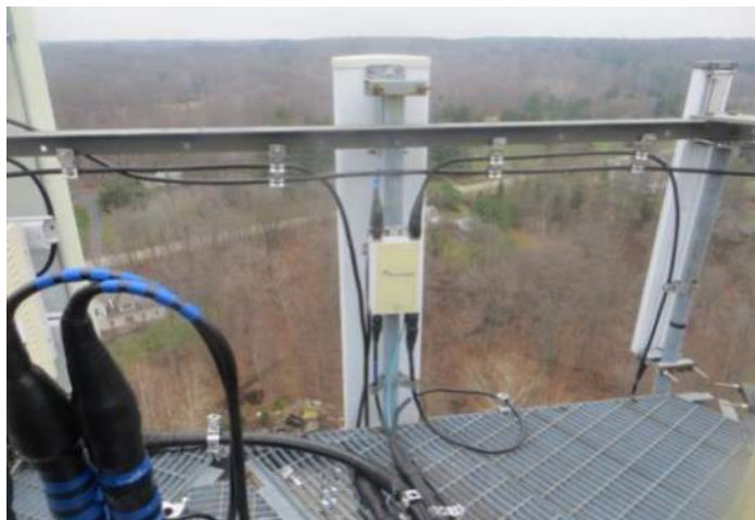
Back Side of Full Ant. #2 (Level & Perpendicular)
