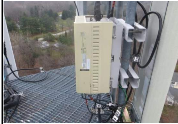
Full Side RRH #1 (Level & Perpendicular)
