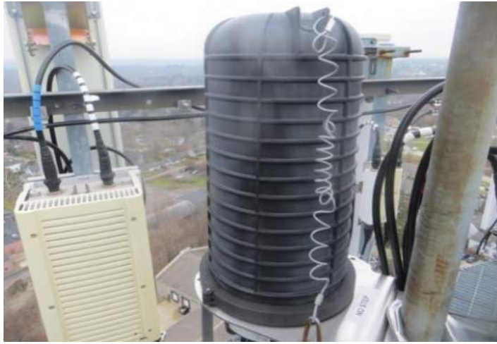
Back Side of Full Surge Protector (Level & Perpendicular)
