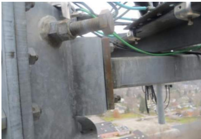
Front Connection at Tower (Level & Perpendicular)
