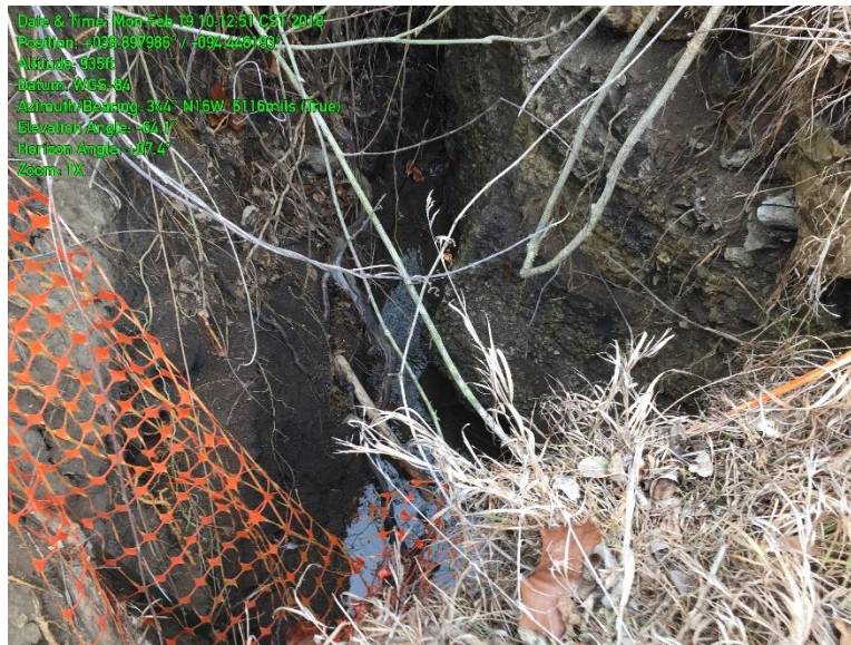
Photo 7- Seepage under emergency spillway
