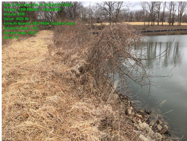
Photo 3- Looking west at freeboard erosion of embankment
