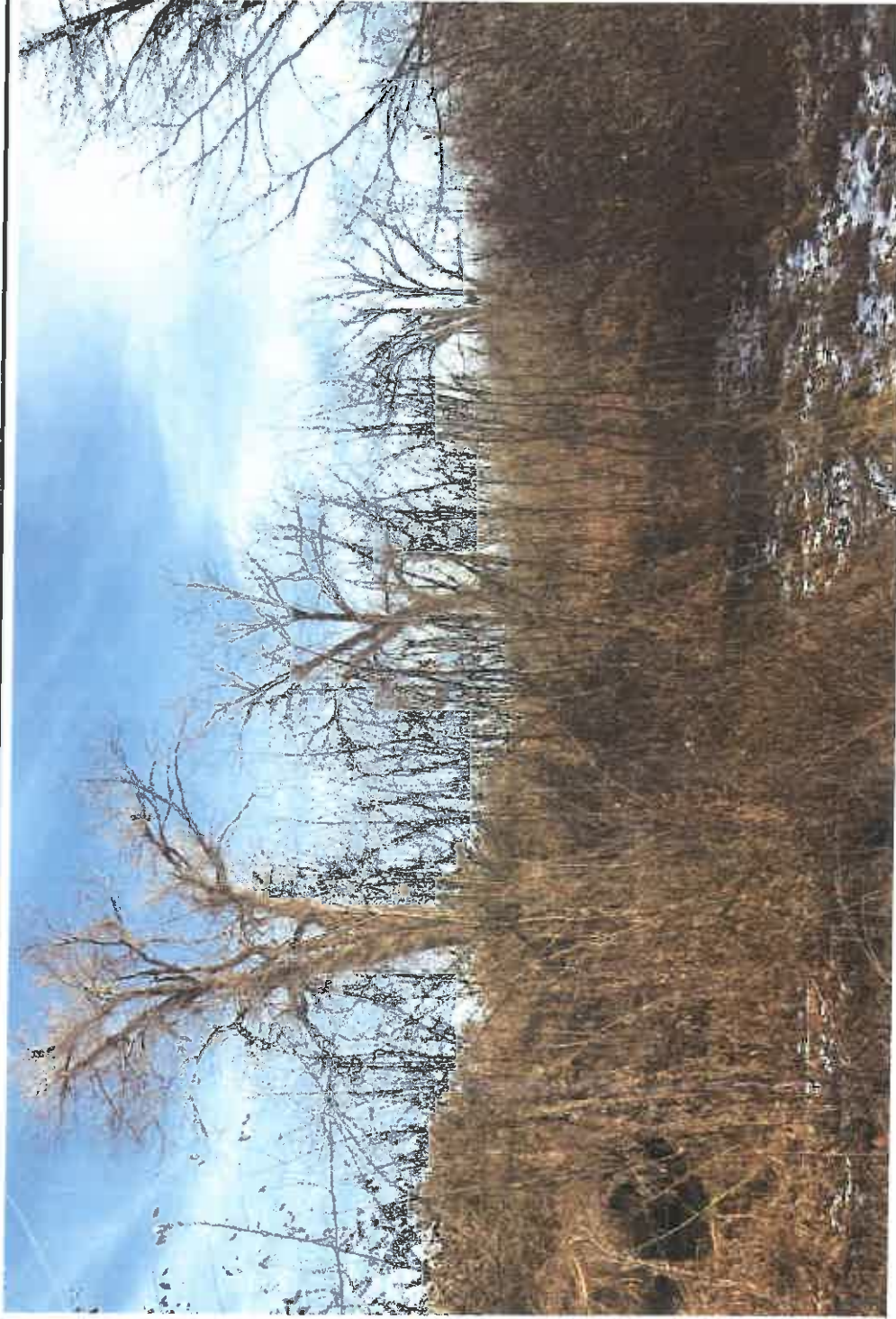
Typical view of woody growth on downstream face of eastern portion of dam.
