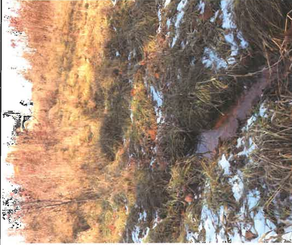
Typical view of water seepage at toe of dam.
