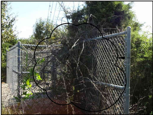
OUTER SOUTH GUY PATH & GUY ANCHOR COMPOUND VEGETATION INTERFERENCE
