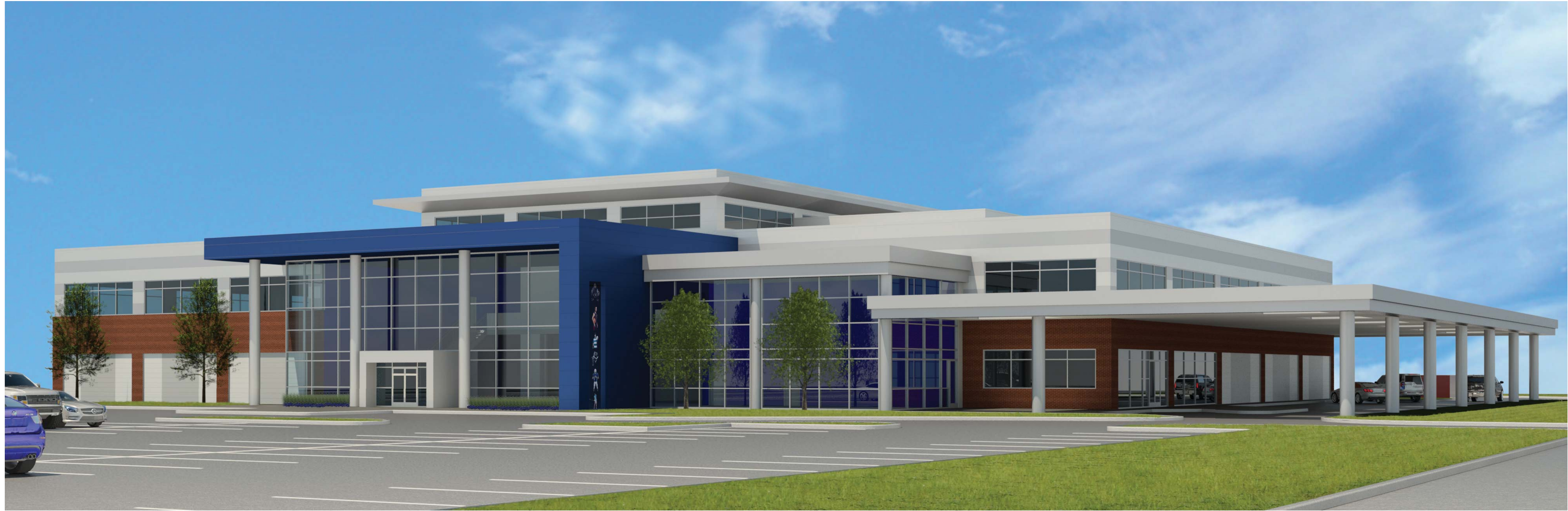
VIEW FROM SOUTHEAST LOOKING NORTHWEST
