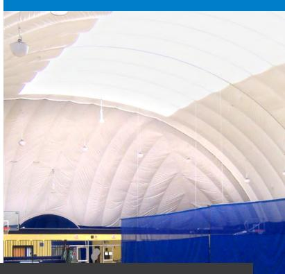
THE ARIZON SKYLIGHT SYSTEM ALLOWS NATURAL LIGHT TO ENTER THE DOME DURING DAYTIME HOURS, SIGNIFICANTLY MINIMIZING OR ELIMINATING THE NEED FOR ARTIFICIAL LIGHTS TO BE ON DURING THE DAY AND RESULTING IN SIGNIFICANT OPERATING COST SAVINGS. THE SIZE OF THE SKYLIGHT IS CUSTOM DESIGNED TO MEET EXACT SPECIFICATIONS.
