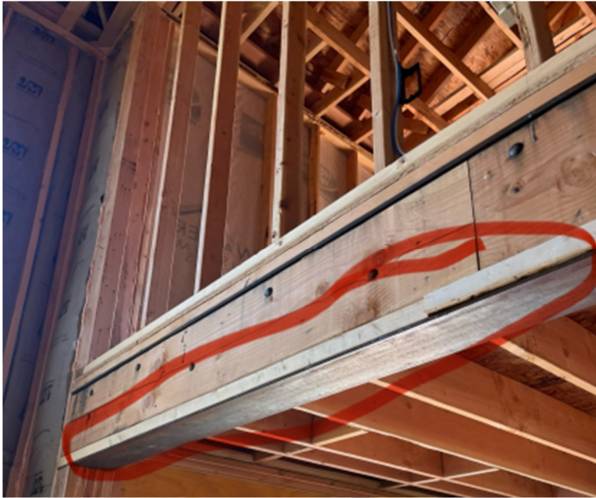
Picture showing installation of through bolts (item #1)
