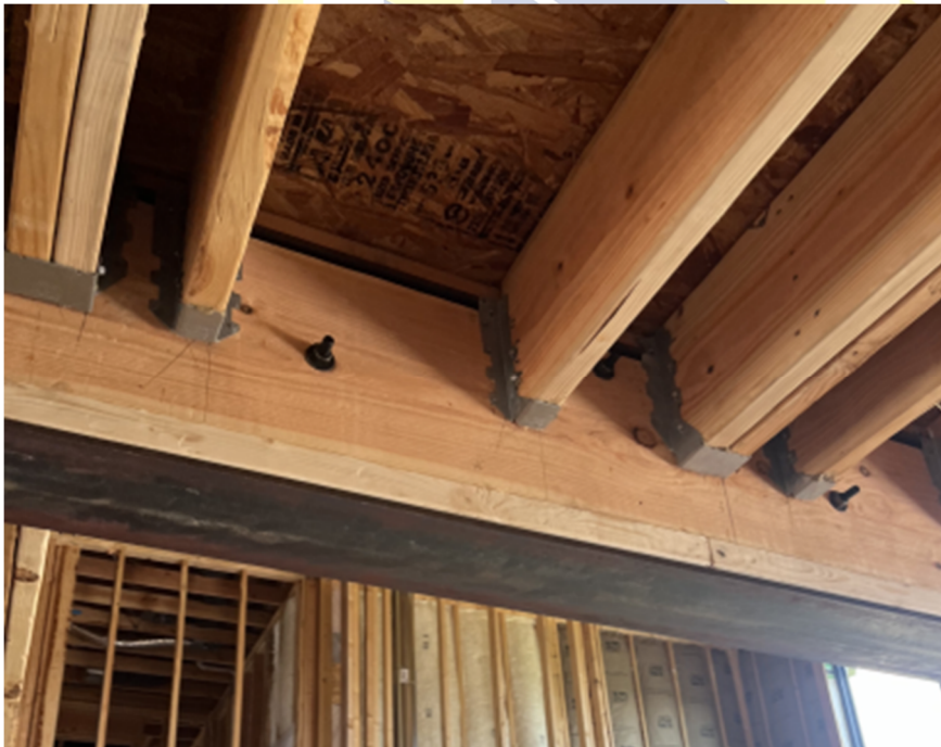
Picture showing installation of through bolts (item #1)
