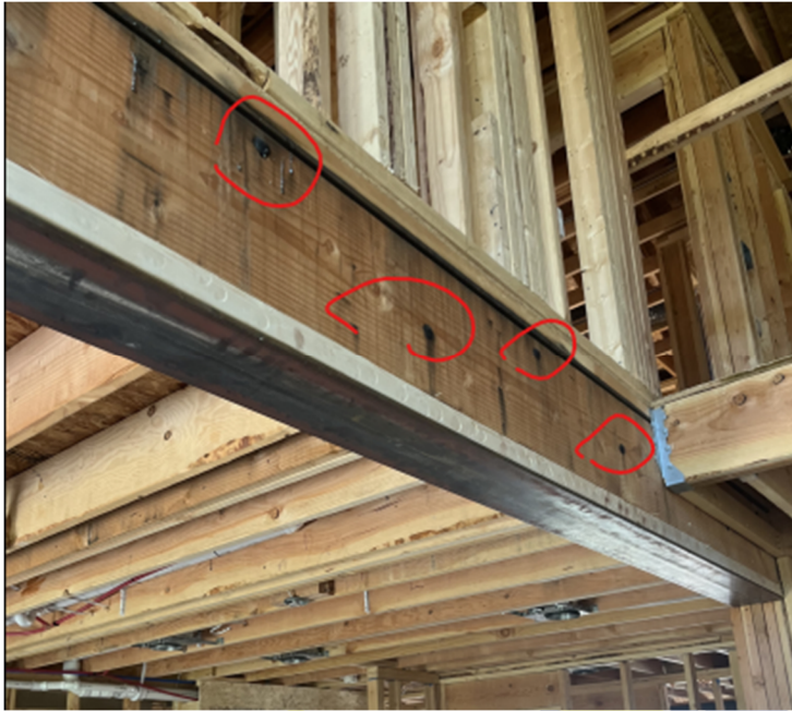
Picture showing installation of through bolts (item #1)
