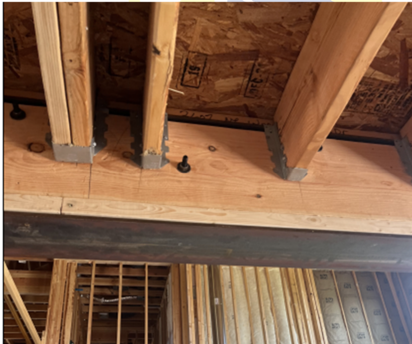
Picture showing installation of through bolts (item #1)
