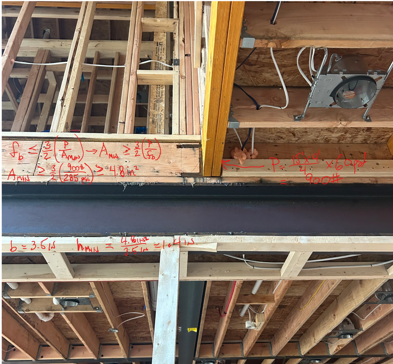
Photo #3 – Connection of beams above W12x50 steel beam
