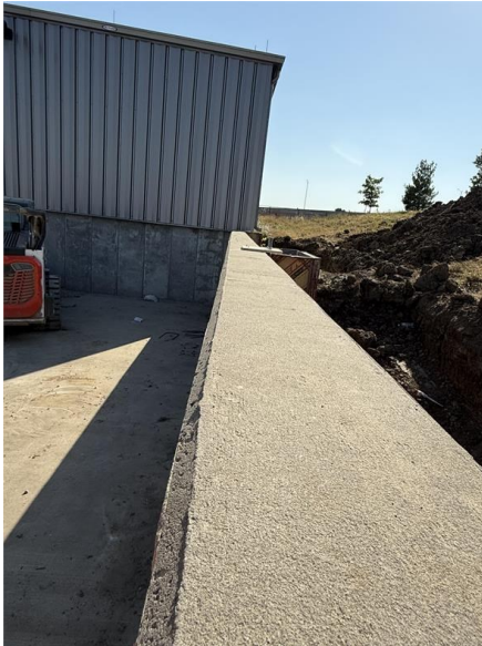
Image Description: 2 pilasters on the West wall
