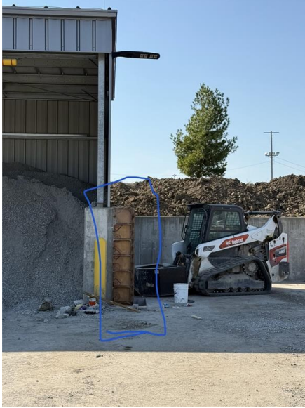
Image Description: SE Pilaster, on the SW corner
