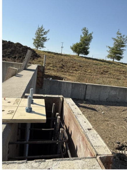
Image Description: Pilasters on the North wall
