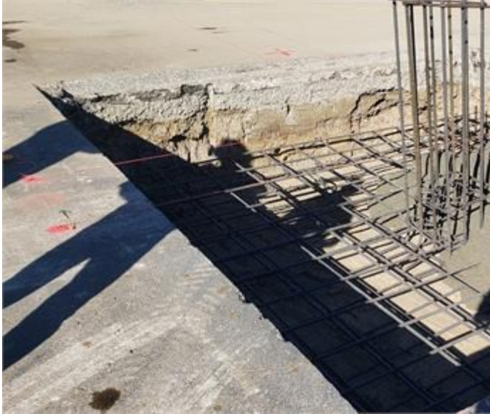
Image Description: SW. canopy footing
