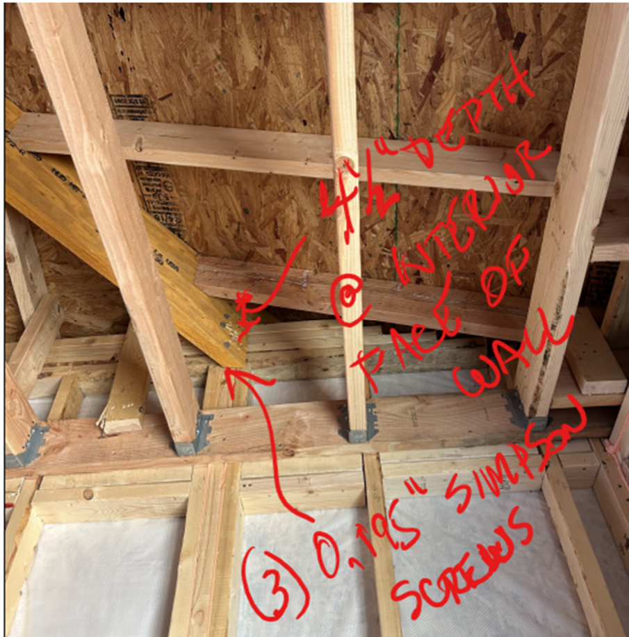
Figure 1 - Overnotched LVL hip
