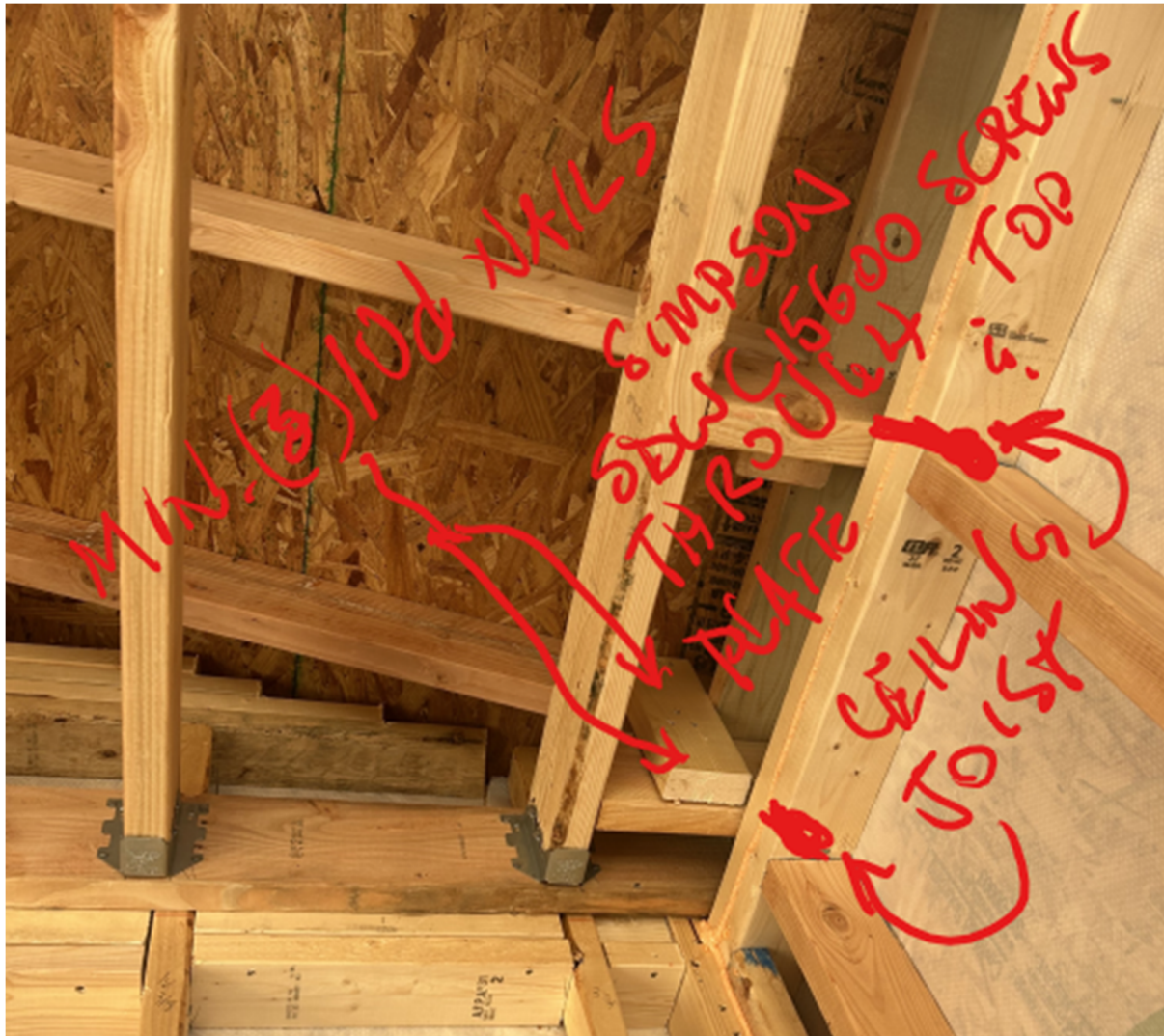
Figure 3 – Top plates not tied together
