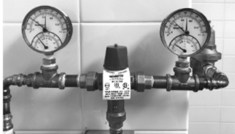
Example of combined temp/pressure gauges and mixing valve
