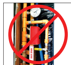
INCORRECT (No pressure relief valve)
