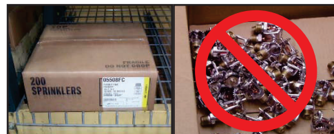
CORRECT (Original container used)
