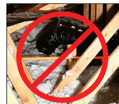
INCORRECT (Exposed piping)
