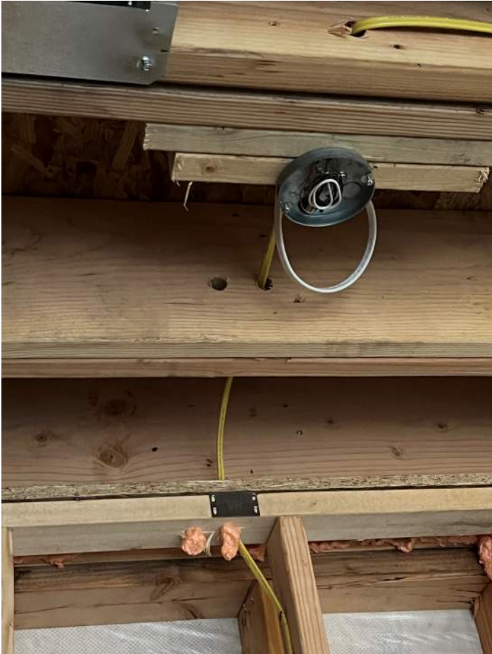
PHOTO 8: JOIST PENETRATION IN REC
