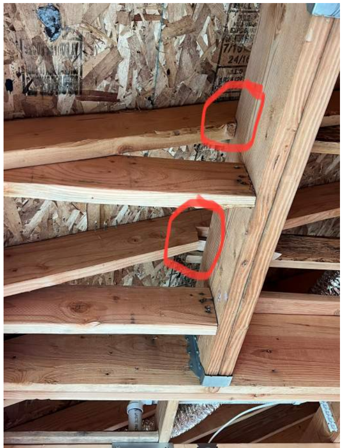
PHOTO 3: RAFTER NOTCH @ MASTER BATH
