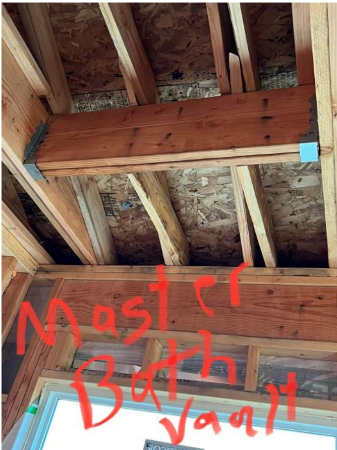
PHOTO 2: RAFTER NOTCH @ MASTER BATH
