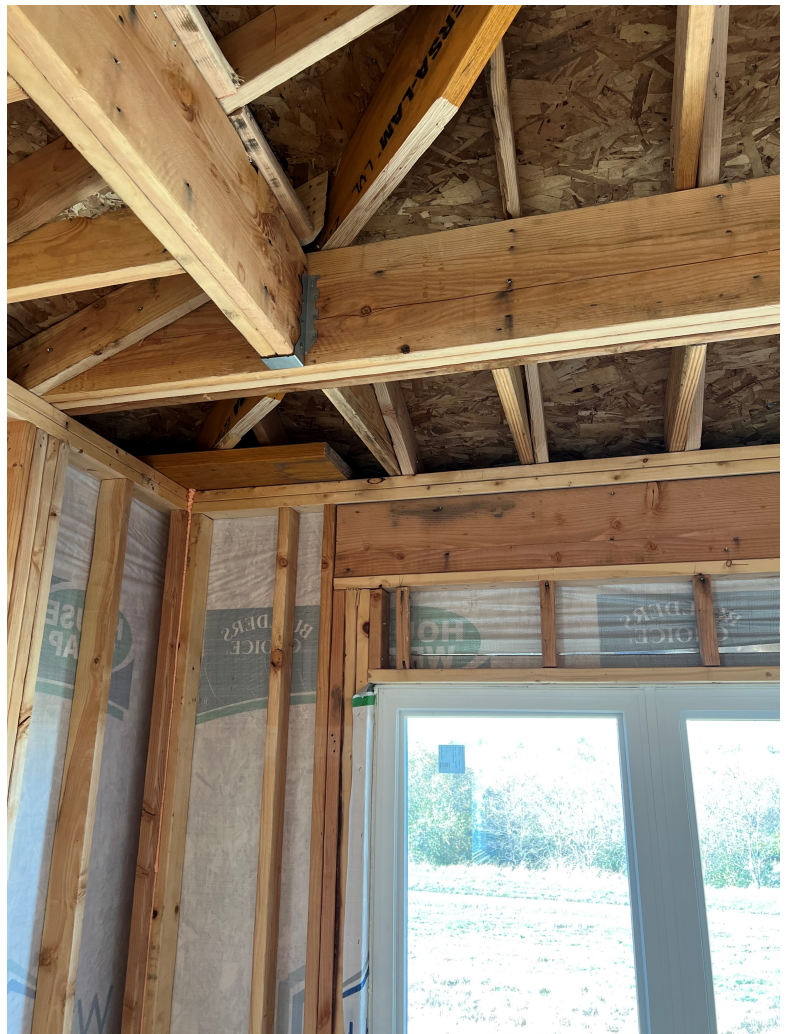
PHOTO 5: HIP RAFTER NOTCH @ MASTER BED
