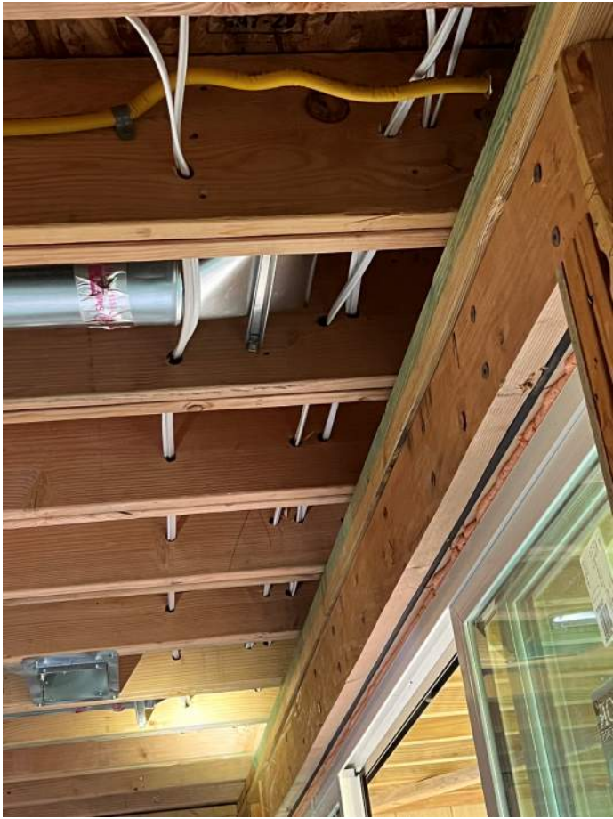
PHOTO 7: JOIST PENETRATION IN REC (ADJACENT TO PATIO DOOR)
