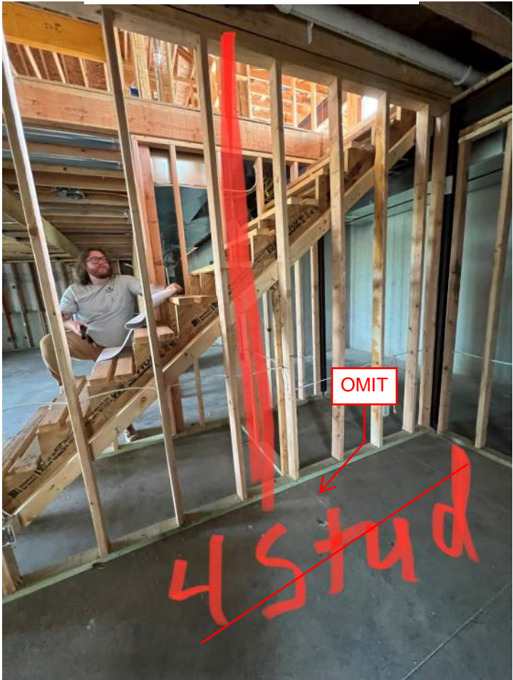
PHOTO 9: OMITED STUD PACK PER PLAN (NO POINT LOAD)
