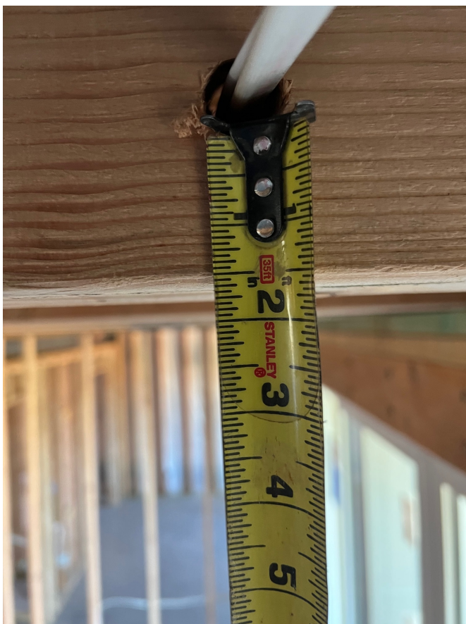
PHOTO 10: JOIST PENETRATION NEAR BOT. OF JOIST (DIM.)
