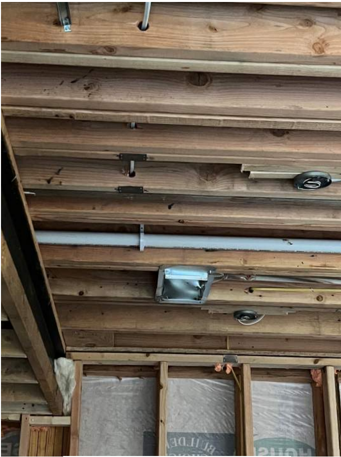
PHOTO 6: JOIST PENETRATION IN REC (ADJACENT TO STEEL BM)
