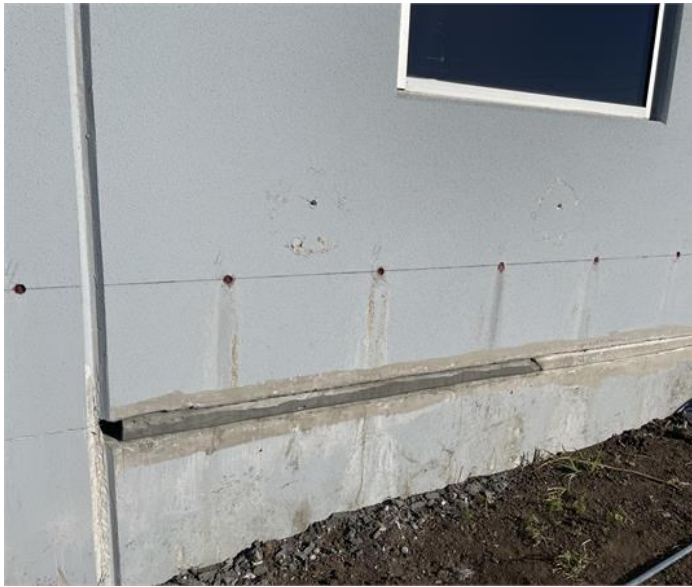
Image Description: Installed anchors
