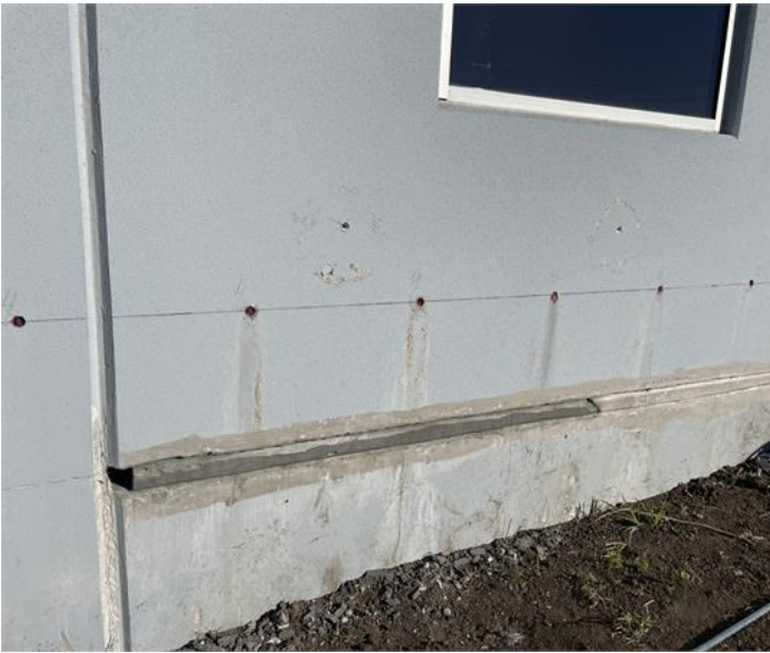
Image Description: Installed anchors
