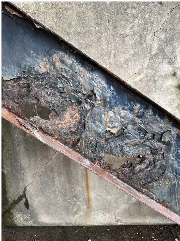
Corrosion of Stair Stringer
