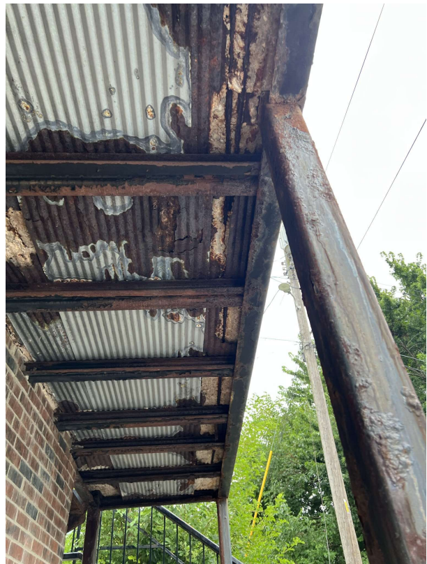
Corrosion of Steel Decking and Transverse Supports
