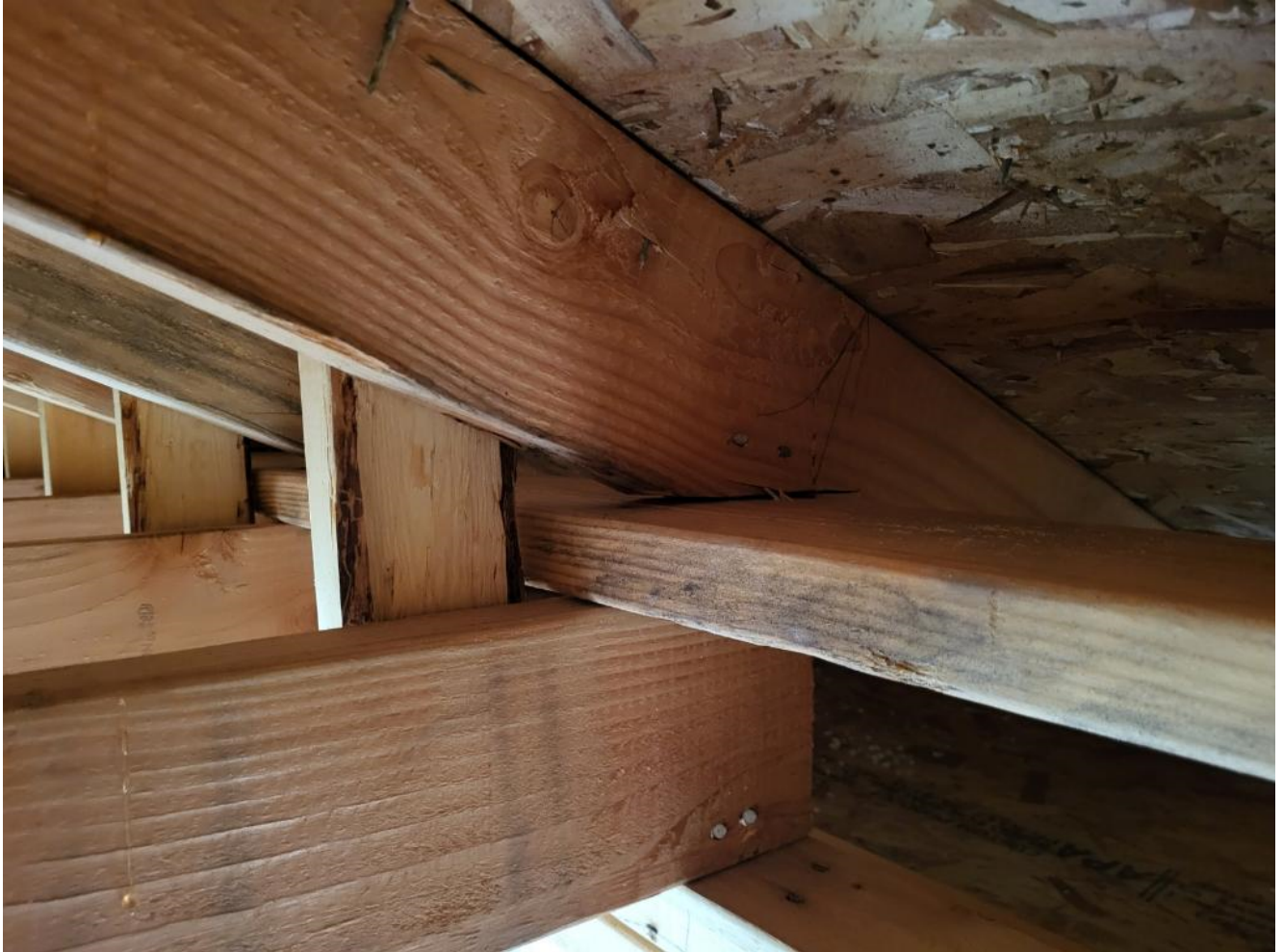
PHOTO 1: RAFTER BEARING CONDITION PER DETAIL 7/S3.0
