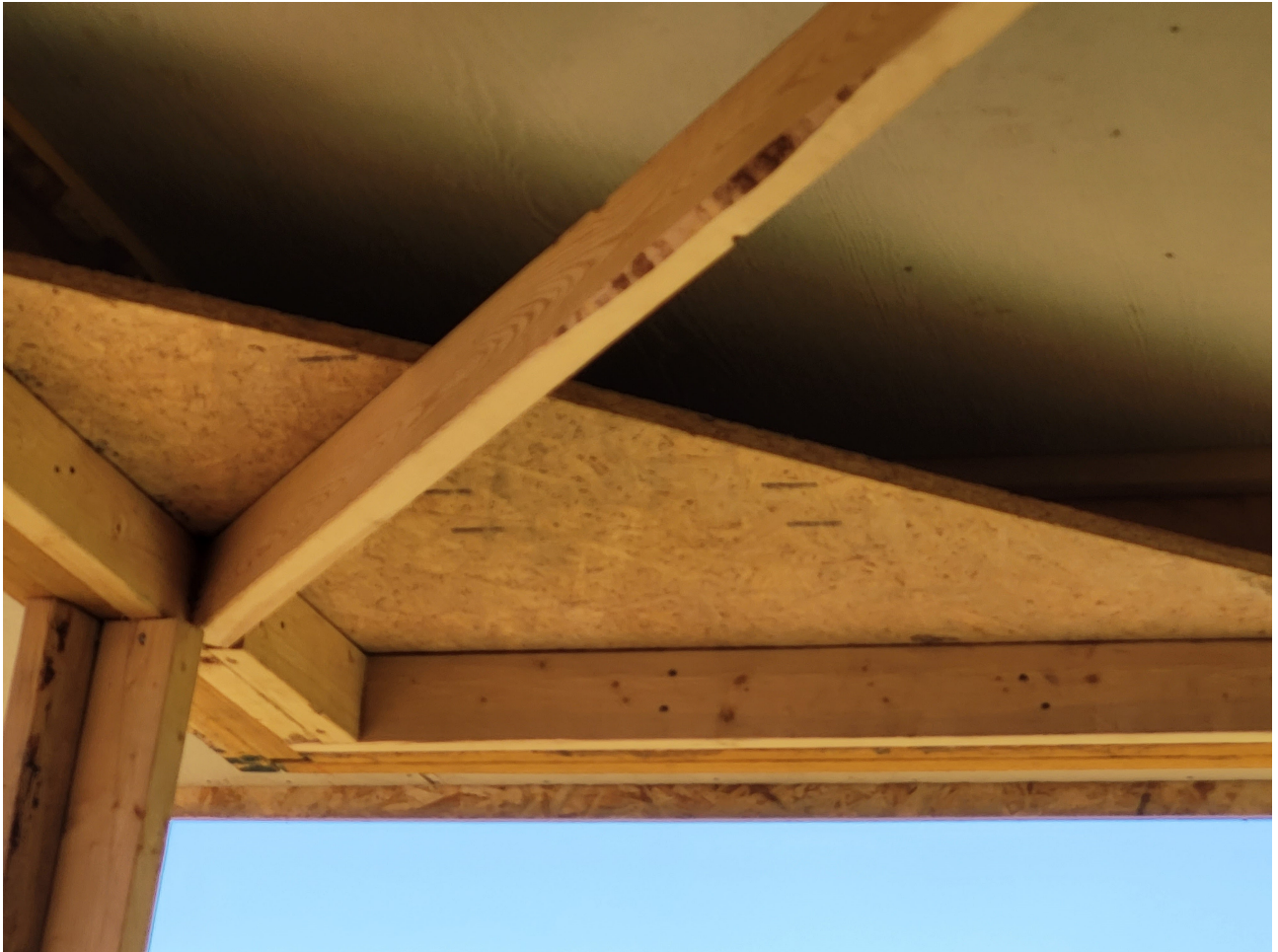
PHOTO 2: END DOUBLE LVL AT BACK PORCH
