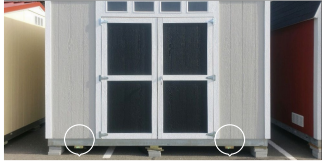
Figure 3 - Display building with wood skids beneath the floor joists
