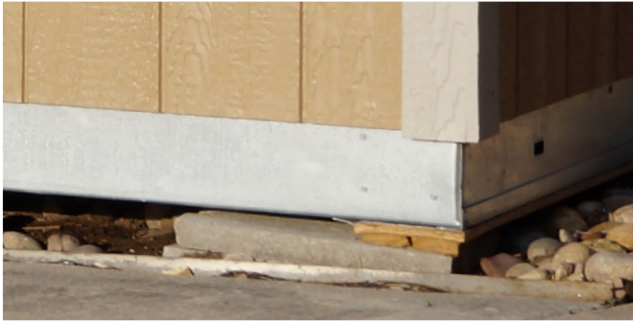
Figure 2 - Close-up of leveling with blocks & shims
