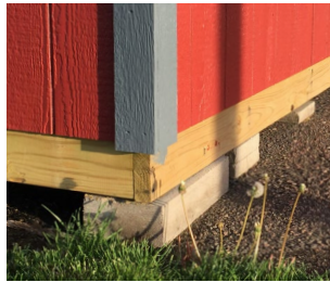
Figure 2 - Close-up of leveling with blocks & shims
