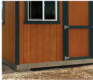
Figure 3 - Display building with wood skids beneath the floor joists
