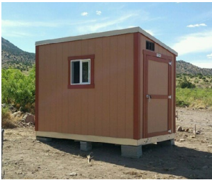
Figure 2 - Close-up of leveling with blocks & shims
