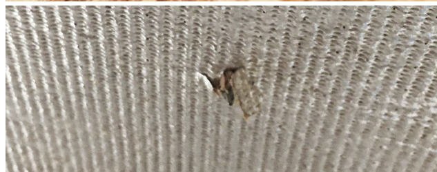
Roofing nails piercing roof decking
