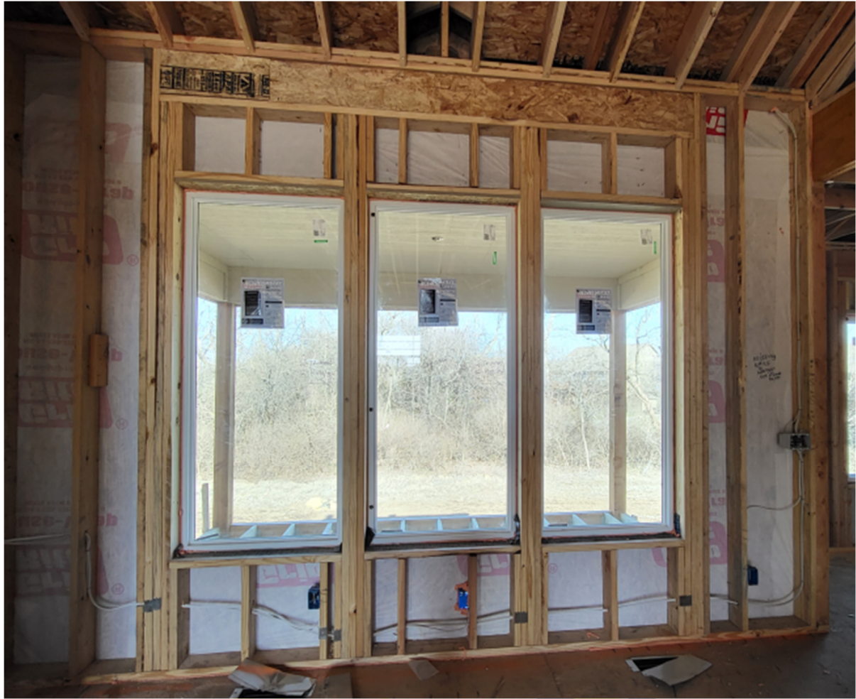
Great room exterior wall framing
