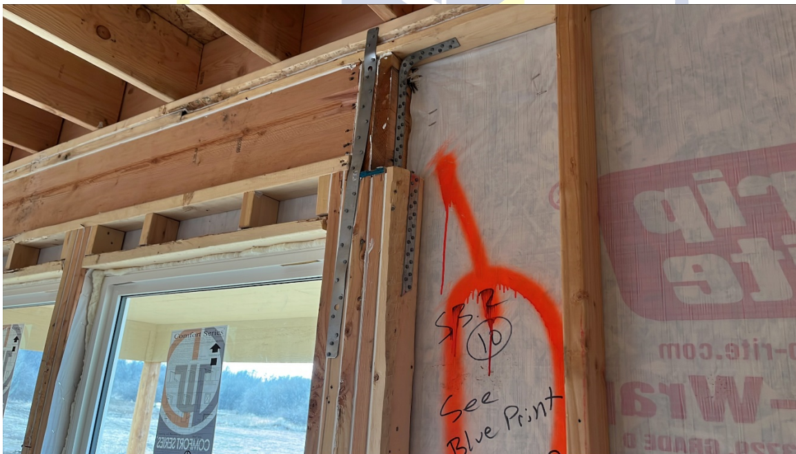
Connection B – header framed into house and attached with strap (right side of covered deck)
