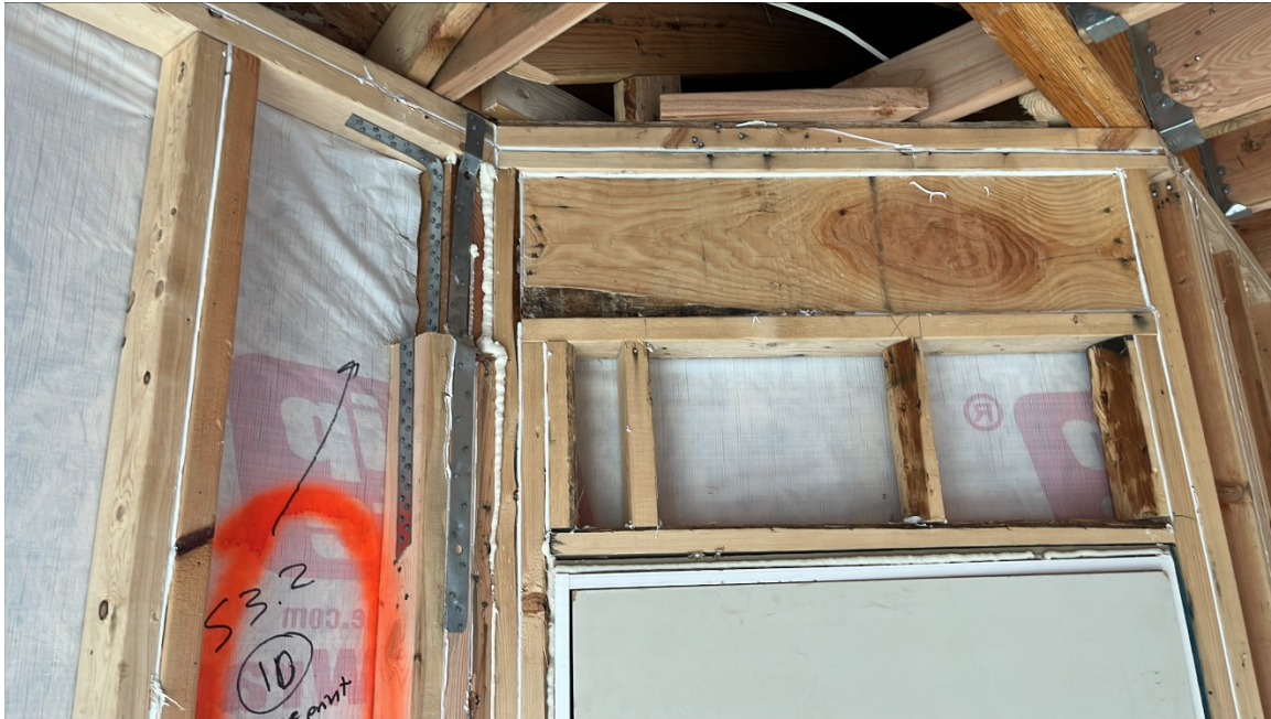
Connection A – header framed into house and attached with strap (left side of covered deck)
