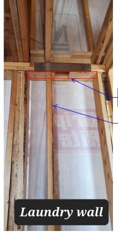
Install 3rd lower 2x top plate with min (6) 10d nails each side of notch.
