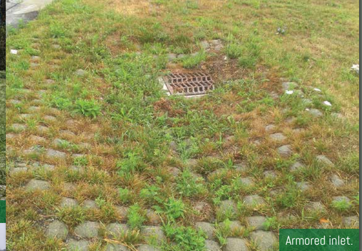
Outlet armored with Flexamat®, 3 years after installation.
