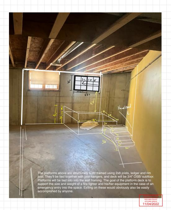
Jat Construct RELEASE FOR CONSTRUCTION AS NOTED FOR PLAN REVIEW 6" r15e 11/04/2022 Steps IIII YUN 246 Joists 2 x le ledger 2 y le rim joist 4x4 Posts 7211 364
