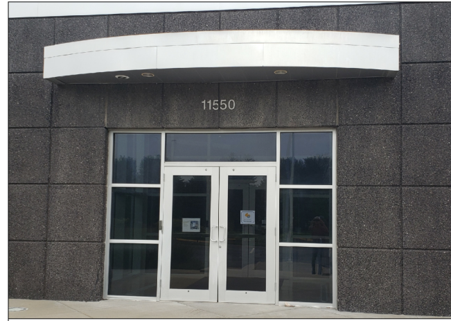
EXPOSED AGGREGATE OMEGA CONCRETE PRECAST INSULATED WALL PANEL COLOR: BLACK GRANITE
