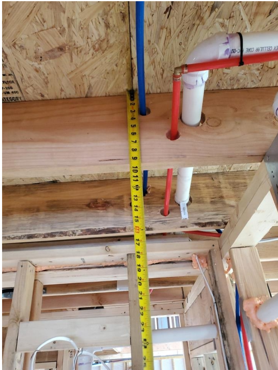
JOIST PENETRATIONS BETWEEN MASTER SUITE/BATH
